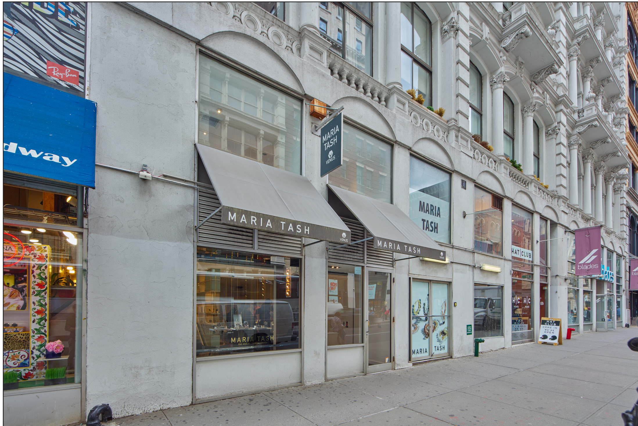
Existing View of 653 Broadway
