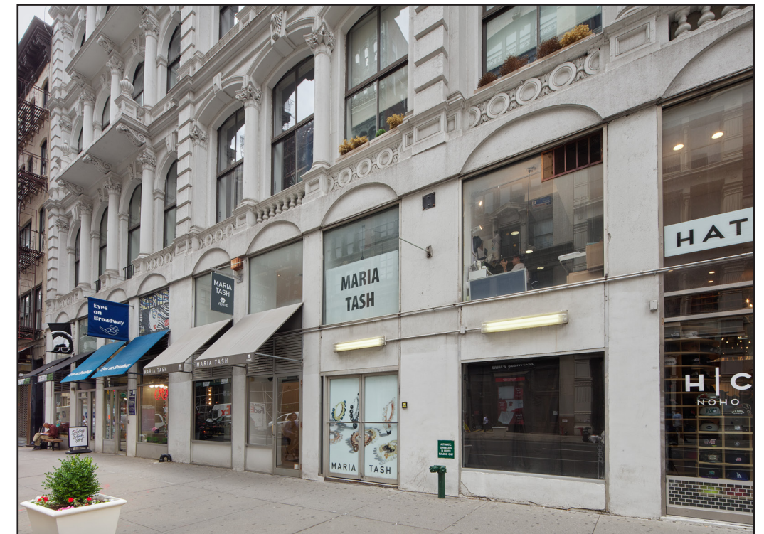
③ Existing View of 653 Broadway Looking South
